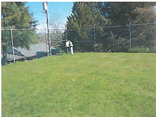
Skyline reservoir vents
