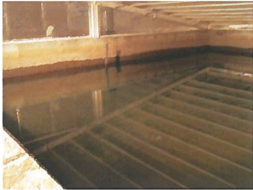
Woodbrook reservoir (roof reflection)
